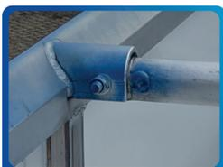
Bolted joint cross beams
